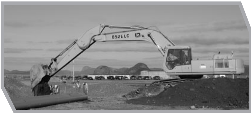
Laying underground piping at the hydromet demonstration plant site
