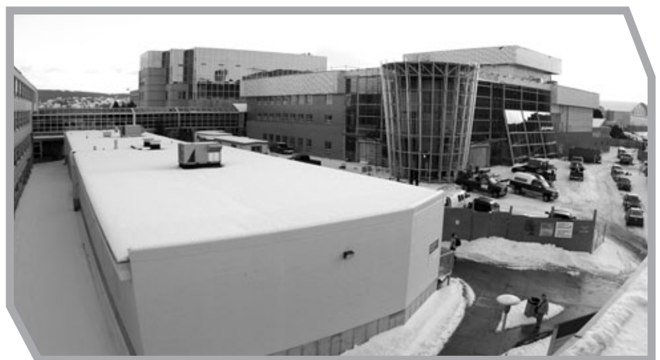
Construction of Inco Innovation Centre at Memorial University
