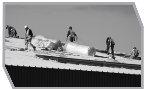
Installing roofing on the process building
