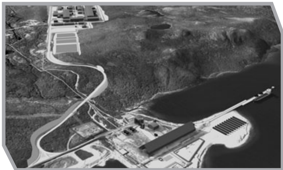
General Layout of the Commercial Processing Plant to be constructed at Long Harbour
