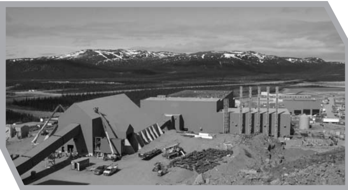
Coarse ore storage building (foreground) and concentrator building
