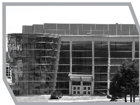
Inco Innovation Centre
