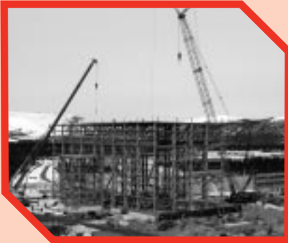
Constructing the Concentrator at Voisey's Bay
