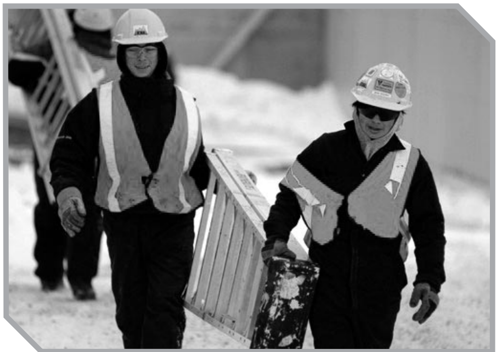
Construction workers at the mine and concentrator site
