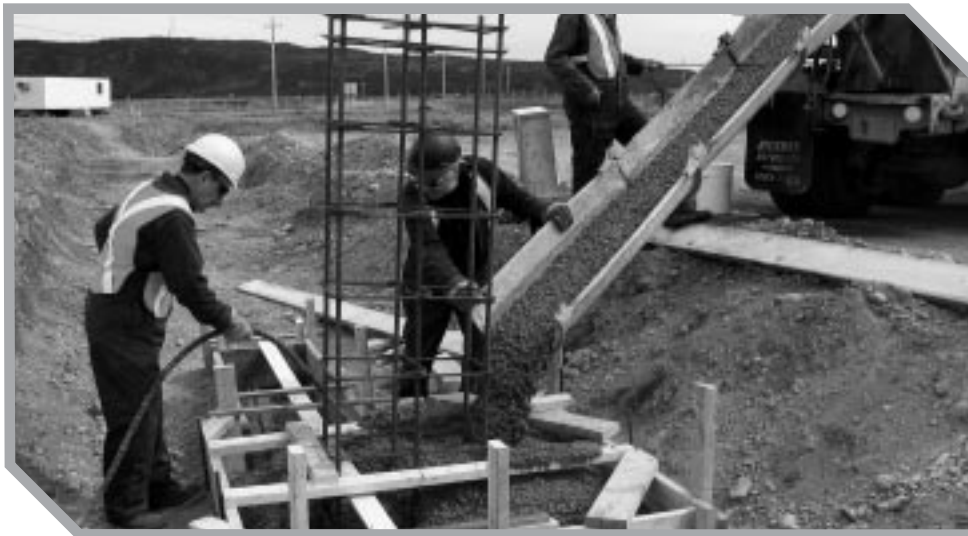
Pouring the first concrete at demo facility site in Argentia.
