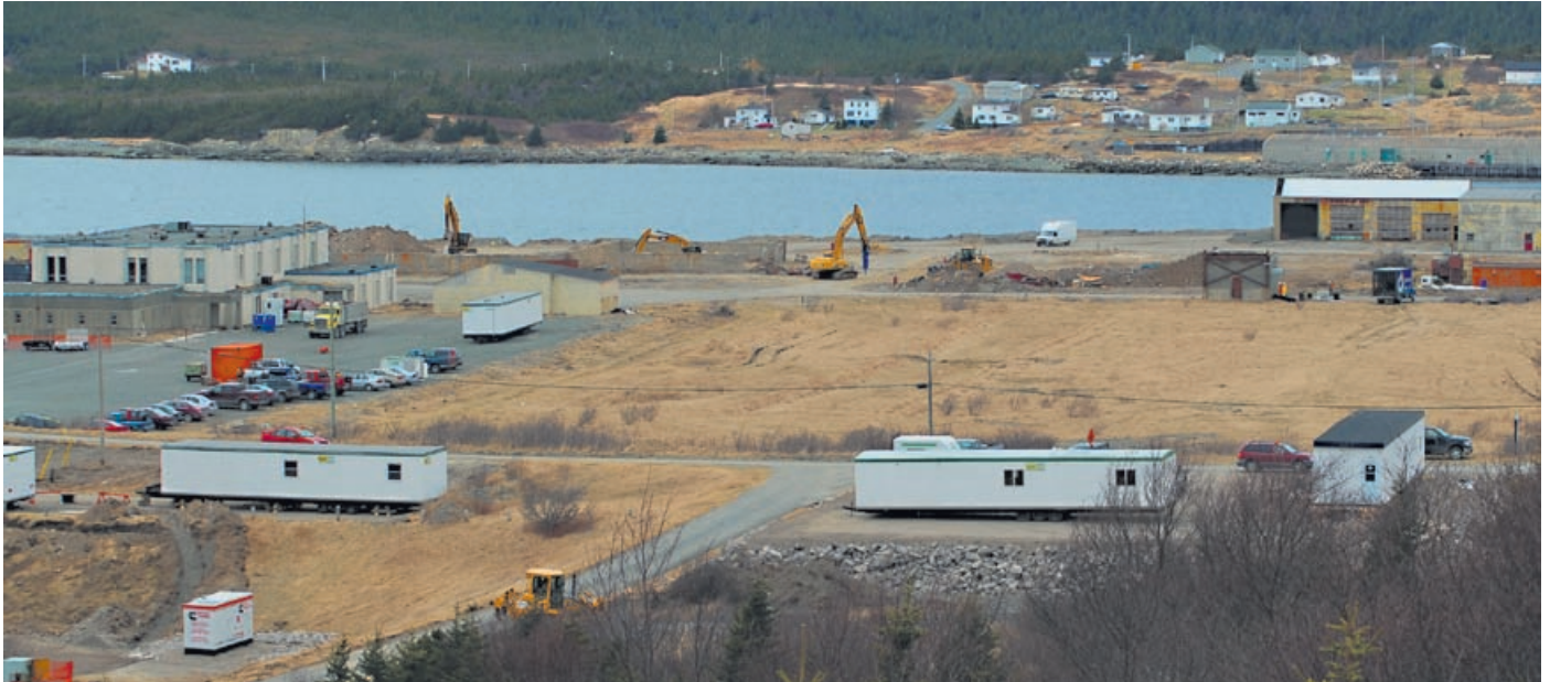
Port Site remediation work at Long Harbour.
