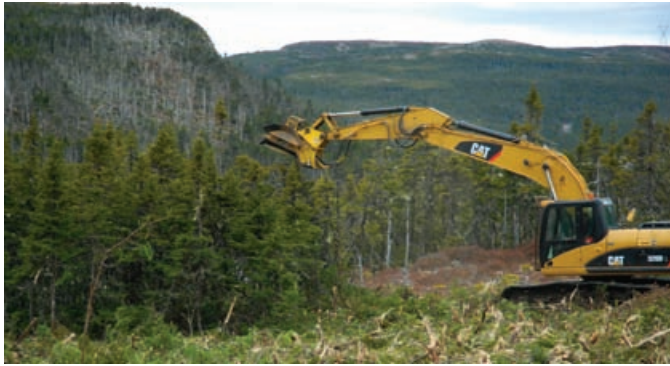
Clearing access road to Plant site at Long Harbour.
