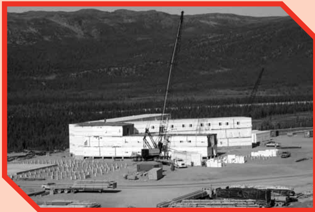
Building the permanent accommodations complex at Voisey's Bay (August 2004)
