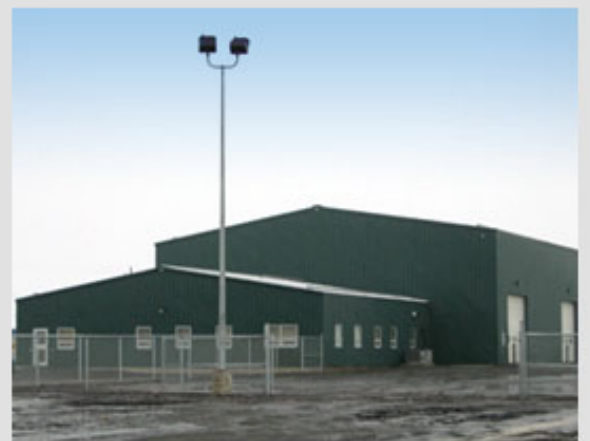
Office/warehouse at hydromet demonstration plant site, Argentia.
